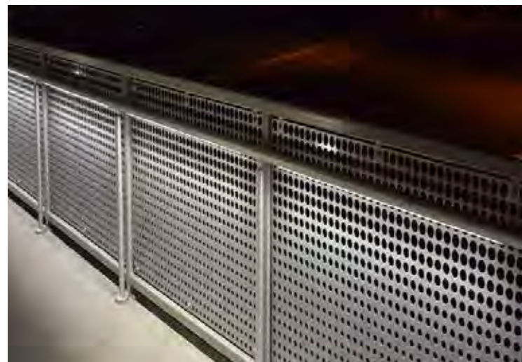
Linear lighting with punched metal infill panels
