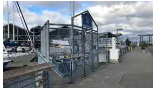
Existing security gates
