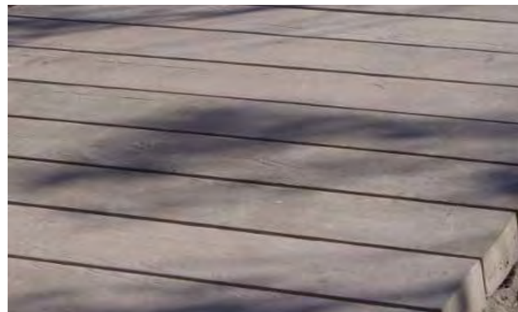
Precast concrete decking
