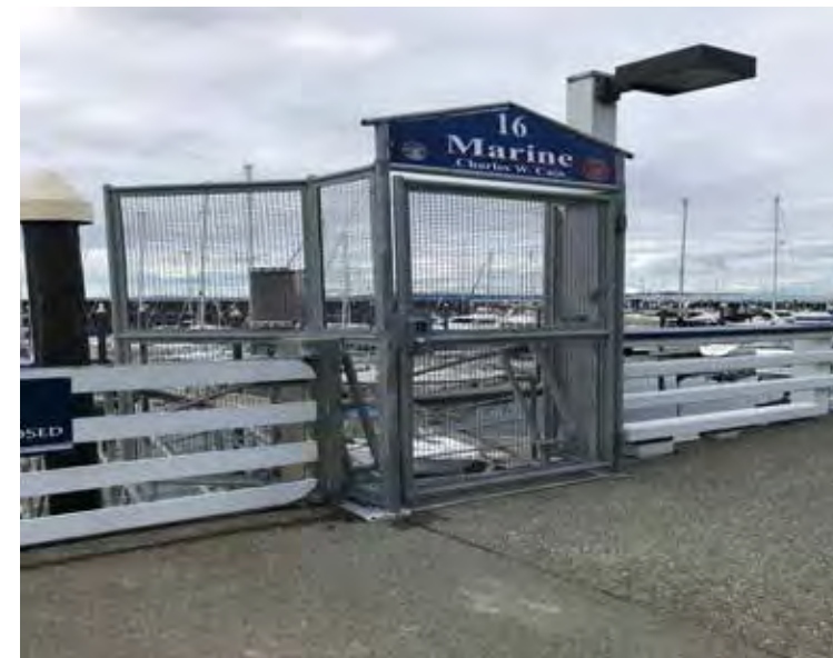
Existing security gates
