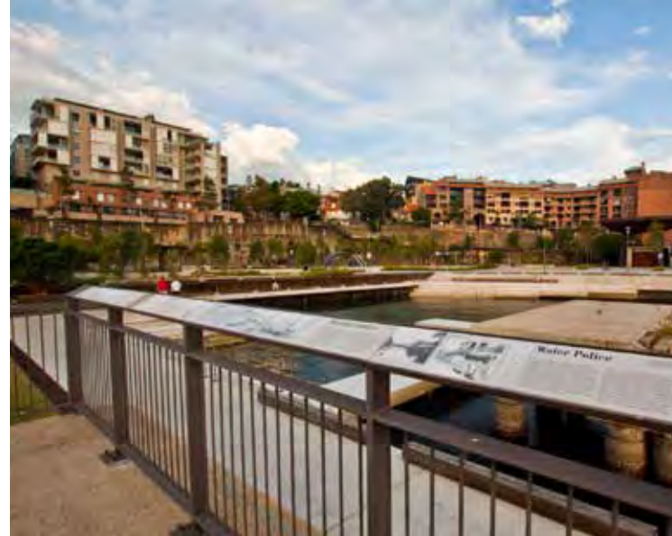
Horizontal interpretive signage integrated into railing
