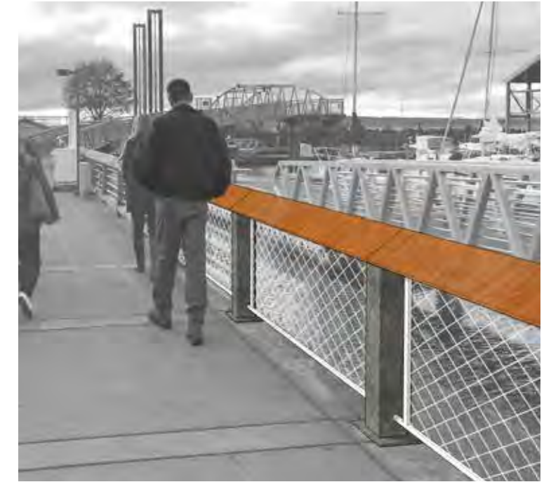
Alternative 3. Existing south Portwalk railing posts with new crimped edge metal mesh panels and new Portwalk rail. Note that central and north railing assemblies would require new post fabrication to match existing south Portwalk posts.
