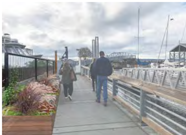
Reduce planter width and move fence back 2.5' to allow for continuous clearance throughout Portwalk.
