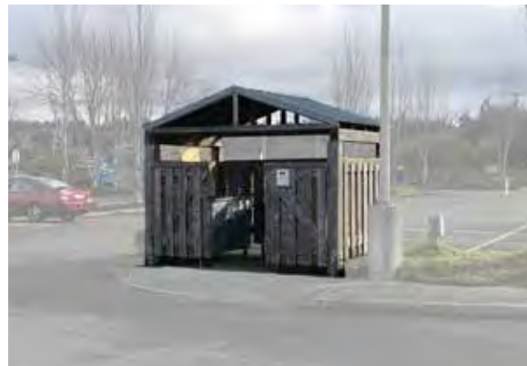
Existing garbage and recycling shelter
