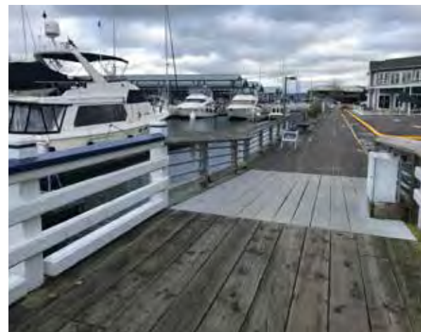
Existing boardwalk surface
