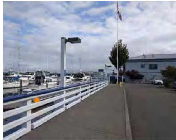
Existing light fixture
