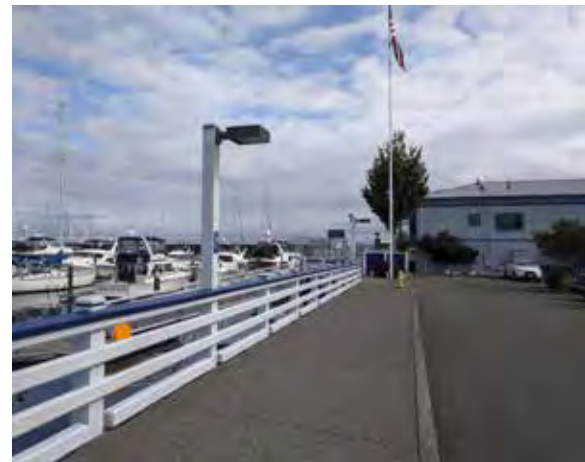
Existing railing designs
