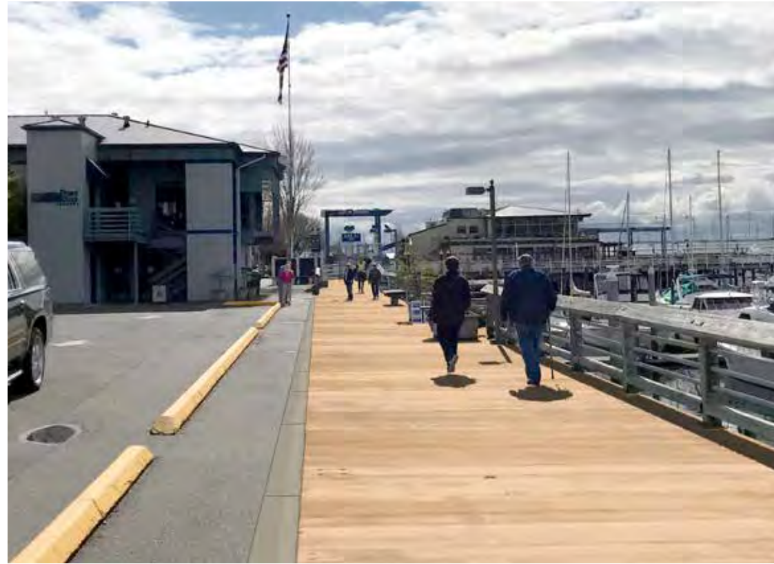
Precast concrete decking
