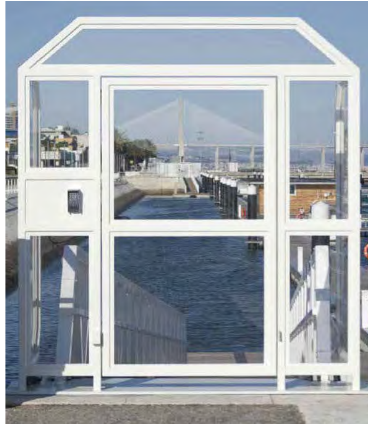
Security gates using transparent glass panels for visibility and a feeling of openness
