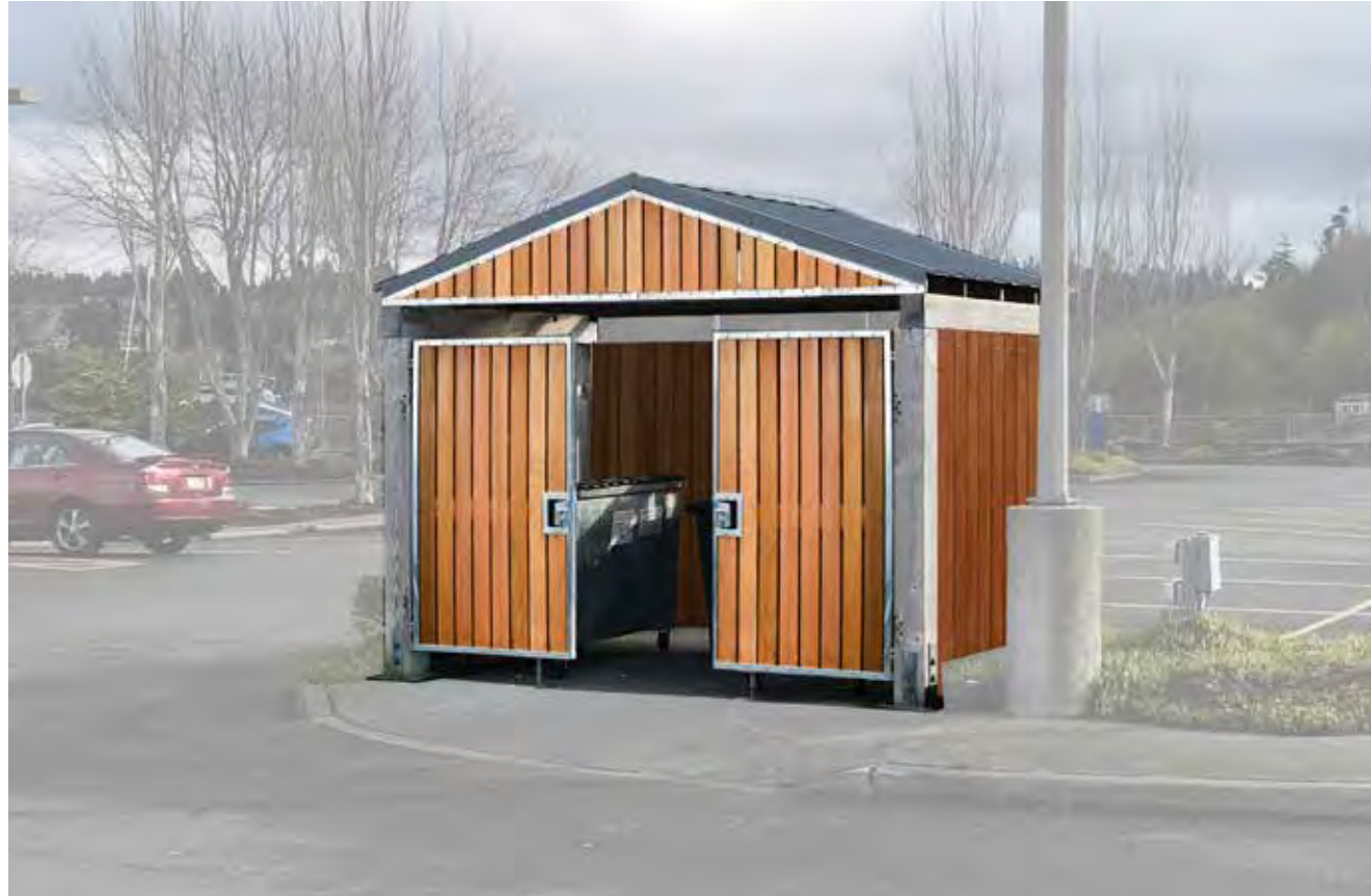
The proposed shelter upgrade replaces the worn wooden slat walls and gates with lower maintenance synthetic materials coordinated with the proposed planters and railing tops.
