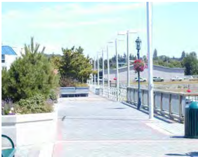
Reorienting the dumpster enclosure and security gates allows for comfortable pedestrian clearance
